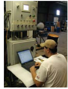
Controls program adjustments
