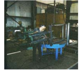
Fabrication of Lance Frame
