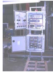
Control & Electrical Panels being wired and tested
